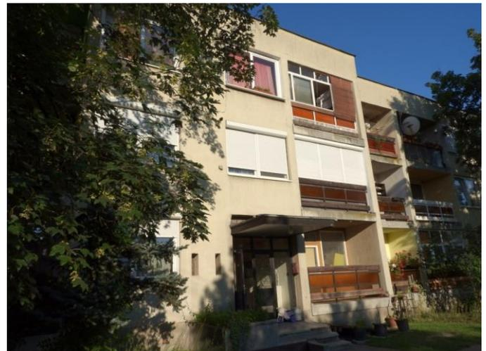
**Figure 1.** Some households in this block suffered from overheating, while others did not – it depended on whether they had external blinds and/or were shaded by the trees. The top floor had problems, but the middle floor pictured here had external blinds so did not face the same issues. (Photo by Neil Simcock)
